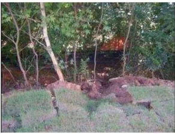
11.5 Item 5(Picture) Rear yard at end of property line
