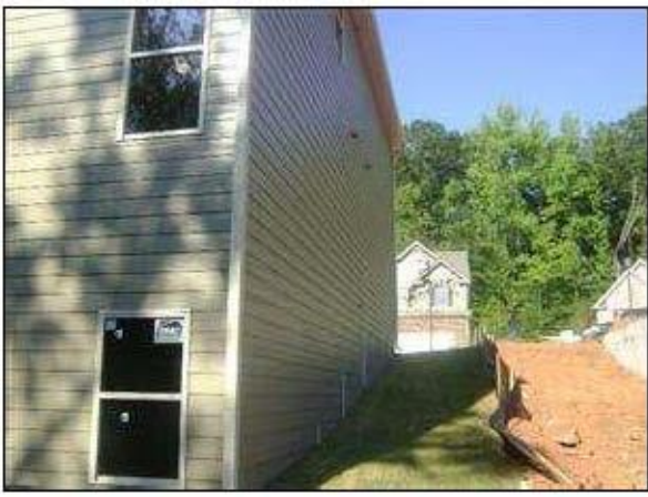
11.0 Item 3(Picture) Side view of home
