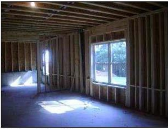
11.5 Item 1(Picture) Basement
