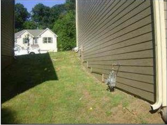
11.0 Item 4(Picture) Side view of home
